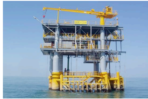
Gambar 1. Wellhead Platform PHE 30 -tipe 4 kaki
